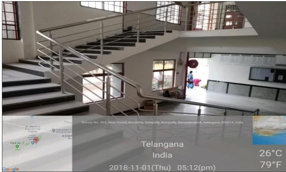
Rail in M.V Block
