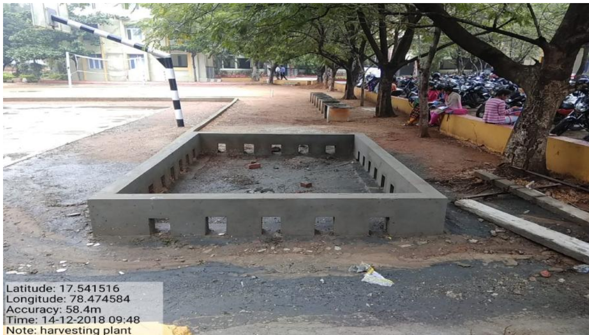
Fig 1(b): Surface Runoff Water harvesting plant in College near parking area
