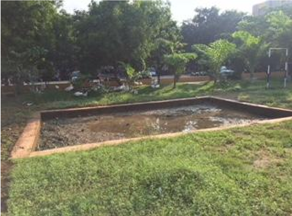
Pic:Water harvesting plant in College Playground
