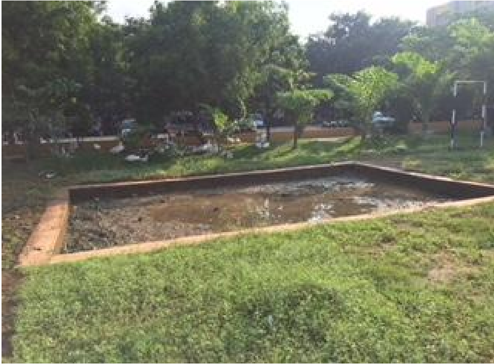
Pic:Water harvesting plant in College Playground
